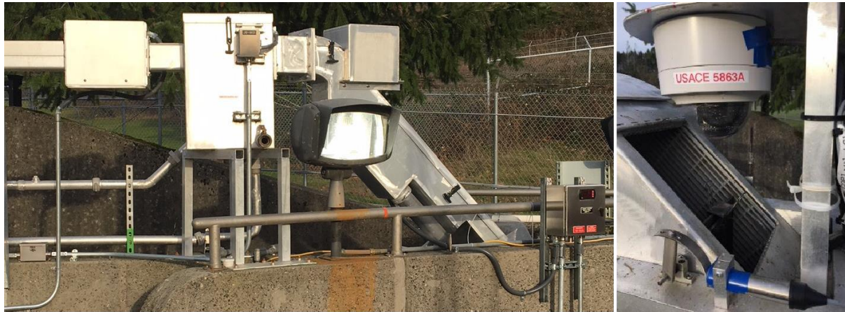
Figure 6. WA-AWS LPS exit showing (left to right) PIT antenna, upwelling box with black latch, camera box (covering the paddle), and Dwyer counter display with red warning tags. Right panel shows camera box with lid removed, globe camera, and proximity detector with blue tape pointed at curved ferrous tab indicating position of paddle (open/closed).
