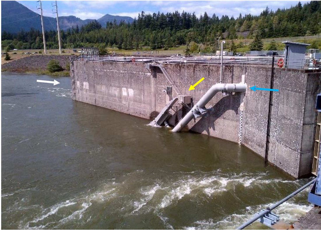
Figure 2. Lamprey Flume Structure (LFS) meets with rest box one (yellow arrow) and attraction water grey pipe (blue arrow) feeds in from below. Washington shore's north upstream fishway entrance at right and north downstream entrance (white arrow).
